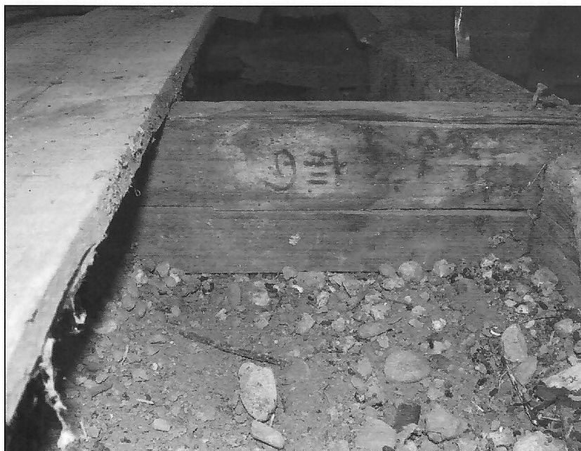
Original Chinese writing was discovered on the fitted floor joists.
