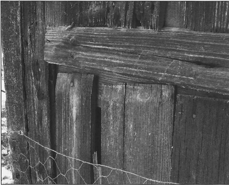
Shrinkage of the fitted joints required supplemental nails, not intended as an original requirement.
